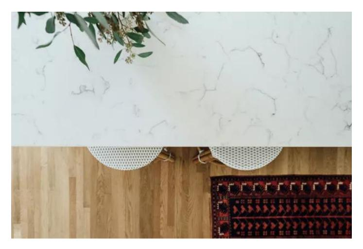
Floor: New and old flooring meet under the island where a wall once existed. Because the original hardwood floor was old and shallow, a cabinetmaker planed down each board individually so that the new flooring could be seamless with the old.
